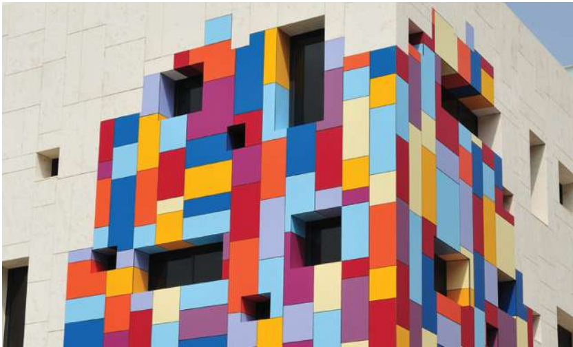
Centro Cultural Ca Don José Canals, Spain Rainscreen façade clad with Trespa Hector Luengo Arquitectos
